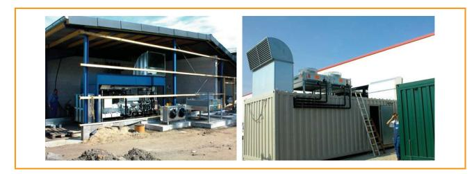
Figure 6.9: Installation of a CHP unit inside a building and in a CHP container [Seva Energie AG]
