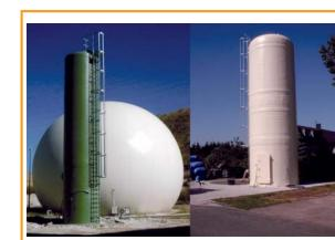
*Figure 6.2: External biological desulphurisation columns, to the right of a gas holder [S&H GmbH & Co. Umweltengineering KG]*
