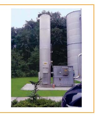
*Figure 3.41: Emergency flare of a biogas plant [Haase Umwelttechnik AG]*
