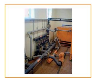
*Figure 3.11: Pumps in a biogas plant* [WELtec BioPower GmbH]
