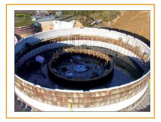
Figure 3.29: A concrete digester under construction [Johann Wolf GmbH & Co Systembau KG]
