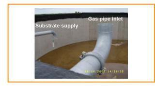
*Figure 3.36: Provisions to prevent disruption of gas extraction; gas pipe inlet with intake opening upward (substrate feed inlet is to the left)* [DBFZ]
