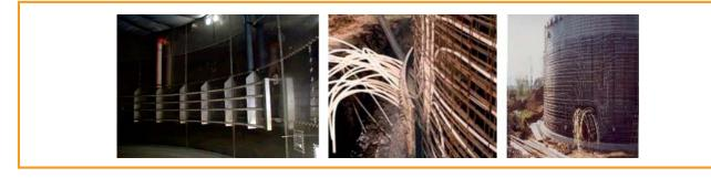
*Figure 3.37: Special-steel heating pipes laid in the digester (inside) (left); installation of heating tubes in the digester wall (right) [Biogas Nord GmbH; PlanET Biogastechnik GmbH (right)]*
