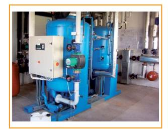
*Figure 6.14: Example of an absorption refrigerator at a biogas plant [DBFZ]*
