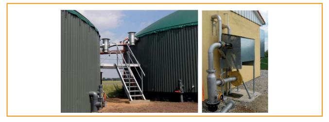
*Figure 3.21:* Working platform between two tanks with piping and pressure-relief devices (left); gas pipe with compressor blower (right) [MT-Energie GmbH (left), DBFZ (right)]
