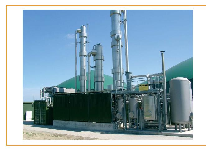
Figure 6.3: Biogas treatment plant (Genosorb scrubbing) in Ronnenberg [Urban, Fraunhofer UMSICHT]
