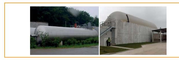
*Figure 3.25: Plug-flow reactors; field examples, cylindrical (left), box section, with overhead gas reservoir (right)* [*Novatech GmbH (left), DBFZ (right)*]
