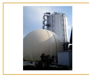
Figure 3.40: Example of a freestanding plastic-sheeting storage tank with two thicknesses of plastic sheeting [Schüsseler, FNR]
