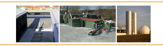
Figure 3.28: Examples of special constructions in dry digestion; sequential batch reactor (left), stirred-tank box digester (centre), methanisation stage of the dry/wet digestion process and external gas storage tank (right) [ATB Potsdam (left), Mineralit GmbH (centre), GICON GmbH (right)]
