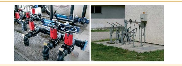
Figure 3.20: Pipes, valves and fittings in a pump station, shut-off gate valves [DBFZ]
