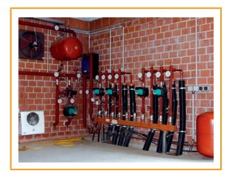
Figure 6.7: Heat distributor [MT-Energie GmbH]
