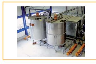
Figure 3.10: Hygienisation with recooling [TEWE Elektronic GmbH & Co. KG]
